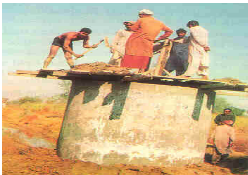
Farmers Participation in construction of Subsurface Drainage Sump
